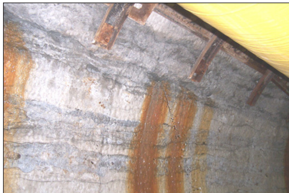
Figure 3. Tunnel sidewall at Station 1+311
